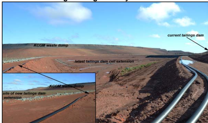
a. New TSF Tailings Storage Facility at Lakewood
