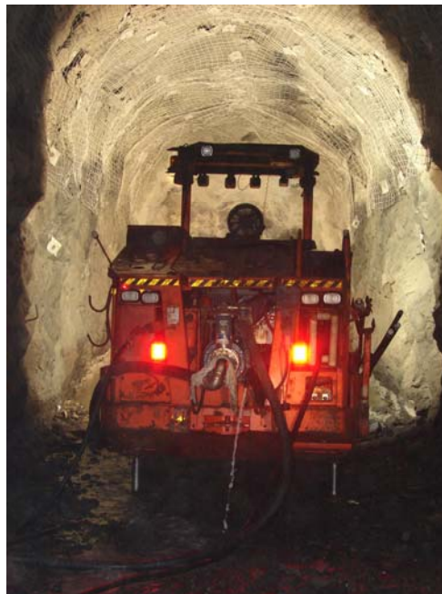
Twin boom jumbo drilling decline face at Daisy Milano
